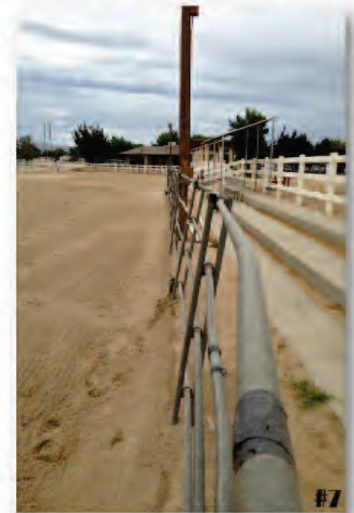
Current Arena Fencing Conditions
